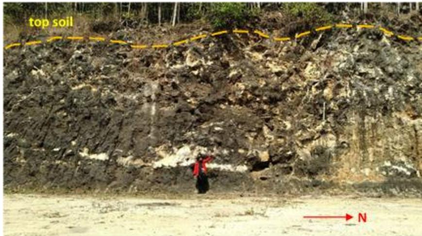
Figure 5. The parking lot in Pindul Cave provided for the tourists is located aside from a steep slope with no engineering that can support the slope stability.
